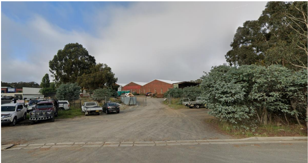
Figure 3– Photo of former Wool Store from Finlay Road
